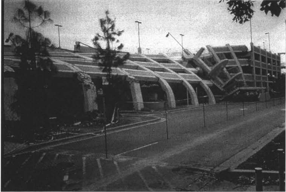
Figure 2.6 Another view of the collapsed parking structure at Northridge [12].
